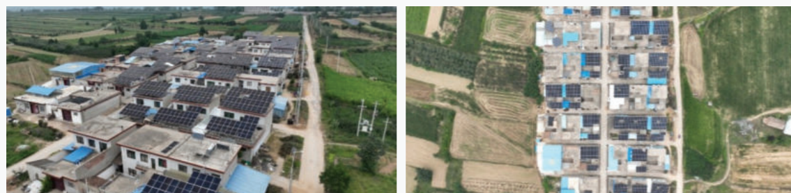
The PV project in Kefang Village, Yaozhou District, Tongchuan City, Shaanxi Province
