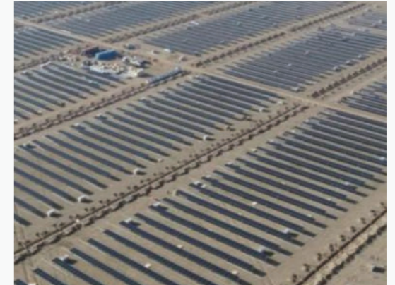
The 1GW solar project in Uzbekistan
