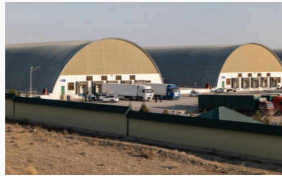
LONGi's PV systems and solutions for humanitarian storage center in Uzbekistan
