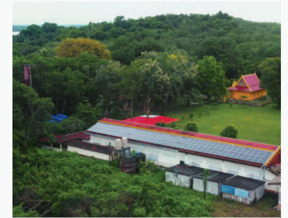
The roof of a Thai resident’s house equipped with LONGi HI-MO solar modules
