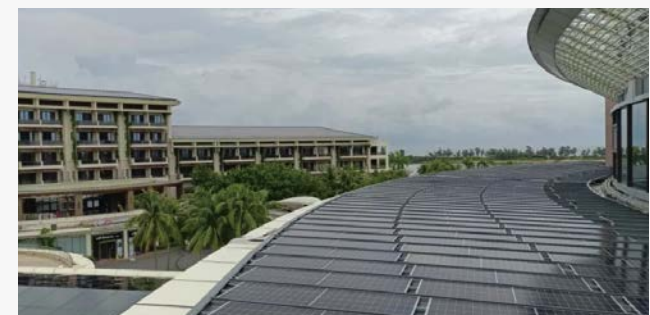
Photovoltaic modules after the passage of a typhoon at level 17
