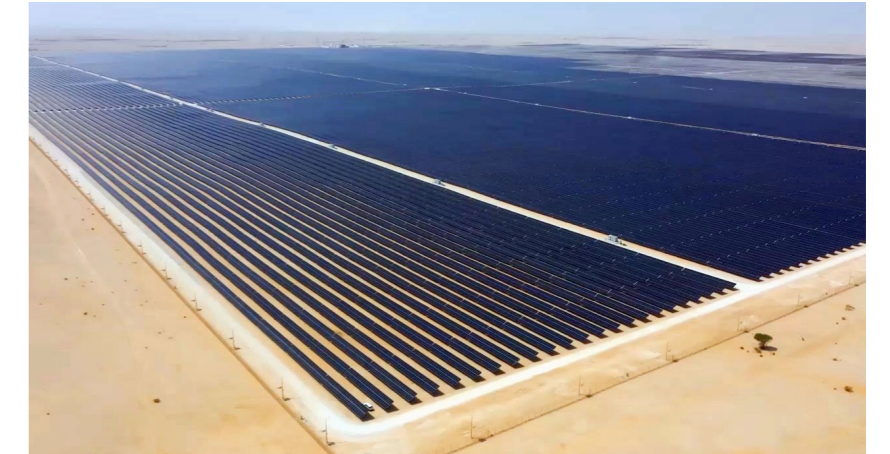
800MW Ground-Mounted Photovoltaic Power Plant in Qatar
