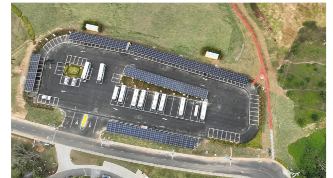
LONGi Park, PV -Storage-Charging Integrated Green Team Station in Boao Zero Carbon Demonstration Zone
