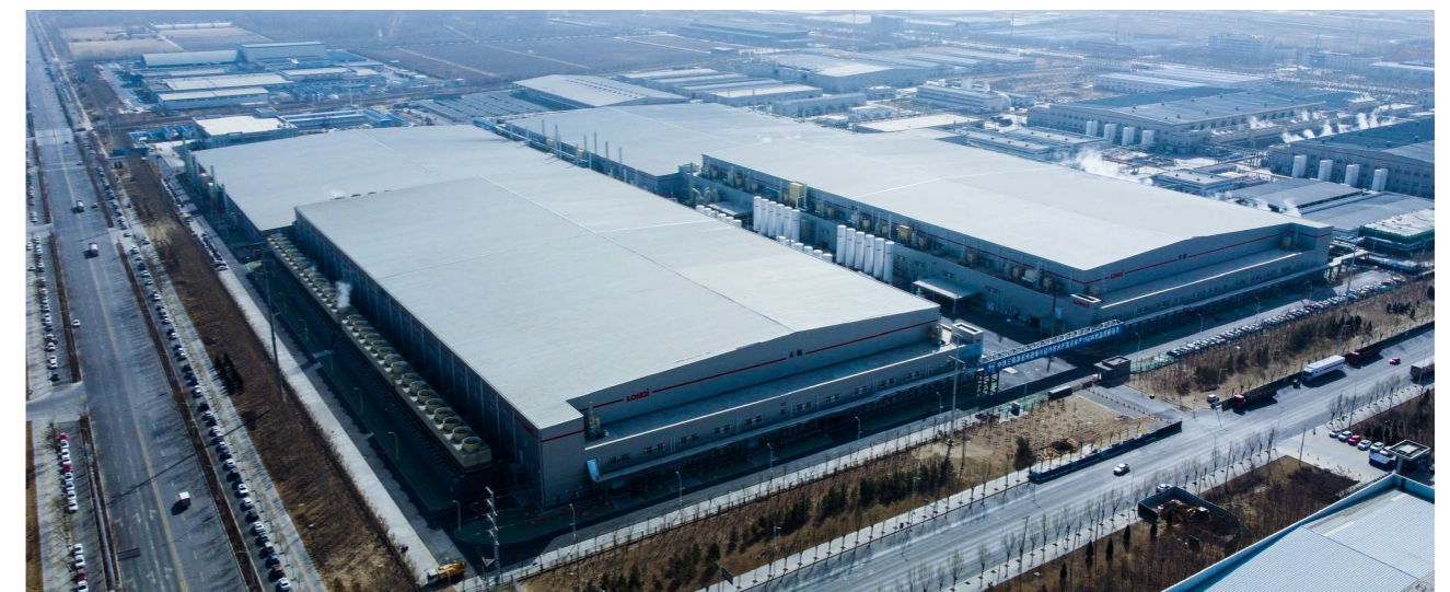
Aerial view of Yinchuan LONGi PV
